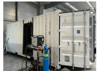
Modifications on a new container
