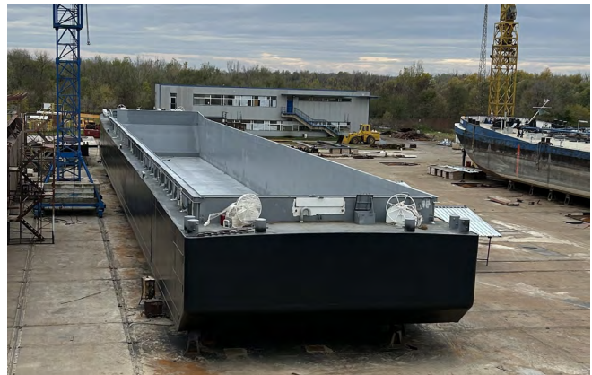
The new Touax 195 under construction
